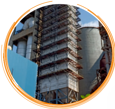
Vertical Cross Flow with Bare tubes for Pre Heater Boiler.
